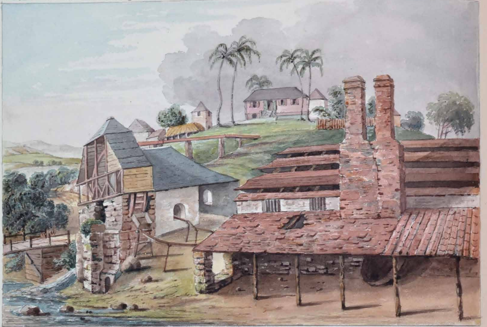
VIEW of the Dwelling, Water Mill, Boiling House &c: taken from station * see Plan page 6.
