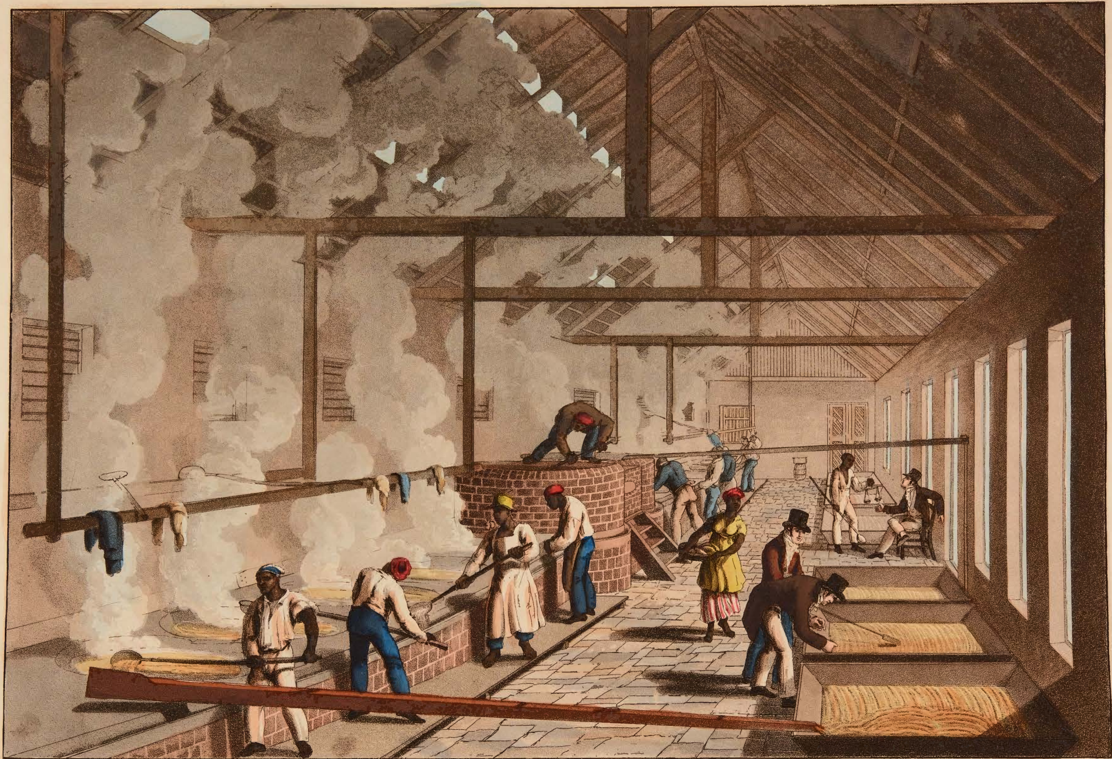
INTERIOR OF A BOILING HOUSE, on Delap's Estate, Antigua.
